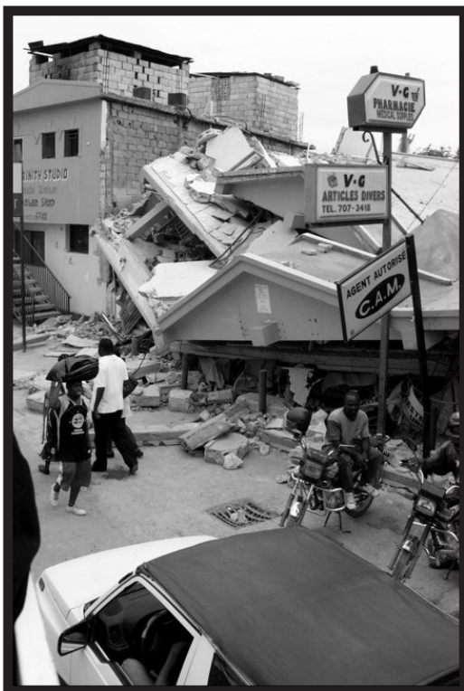
Destroyed shopping district near the orphanage
