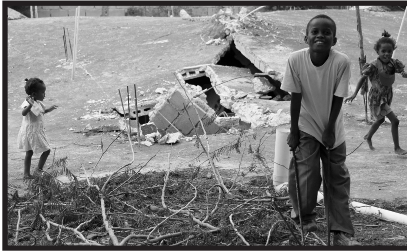
Children playing on the roof of a collapsed building
